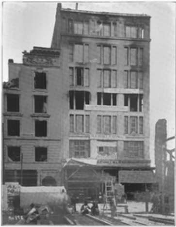
KAMM BUILDING. South side of Market Street, near Third. The facade consists of Colusa sandstone, which remains in first-class condition. The steel center has fallen away. The rear half of this building was wrecked by the failure of columns in the basement story, where a large stock of highly inflammable wall paper furnished fuel for a fire that burned continuously for a whole month. In the front portion of the building, where normal conditions prevailed, the steel skeleton frame and the working concrete floors and walls both and plaster ceiling, remain in their original condition. The building was left and plaster partitions remain standing, but are deluged out of ground in some places. The illustration shows also the half of the front of the Spreckels Building, lower on the left-hand side.
