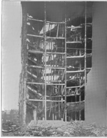
KAMM BUILDING. Showing the collapsed rear portion of the building caused by column failure in the basement. The tenacity of the connections of the wall girders at the entrance is remarkable. Two beams flamed in them, when canted downward in the center, have twisted the girders in the middle section through an angle of about 90 degrees from the vertical. The working concrete floors cling to the beams; seven tiers in the rear of the building being inclined at an angle of about 33 degrees, and other sections of the floors being warped and distorted into almost every conceivable shape. Note the curved skyline of the rear where the central columns have been shown twisted by the collapse.
